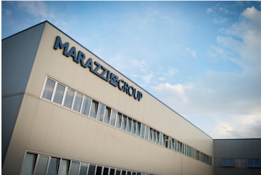
Marazzi Group – Plant of Fiorano Modenese
